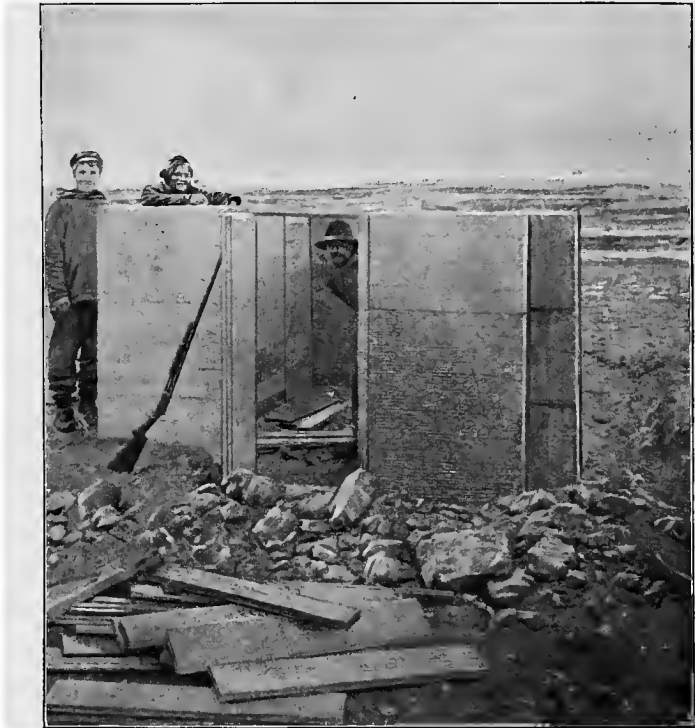
BUILDING THE MAGNETIC VARIATION HOUSE. GJÖAHAVN, 1903.
